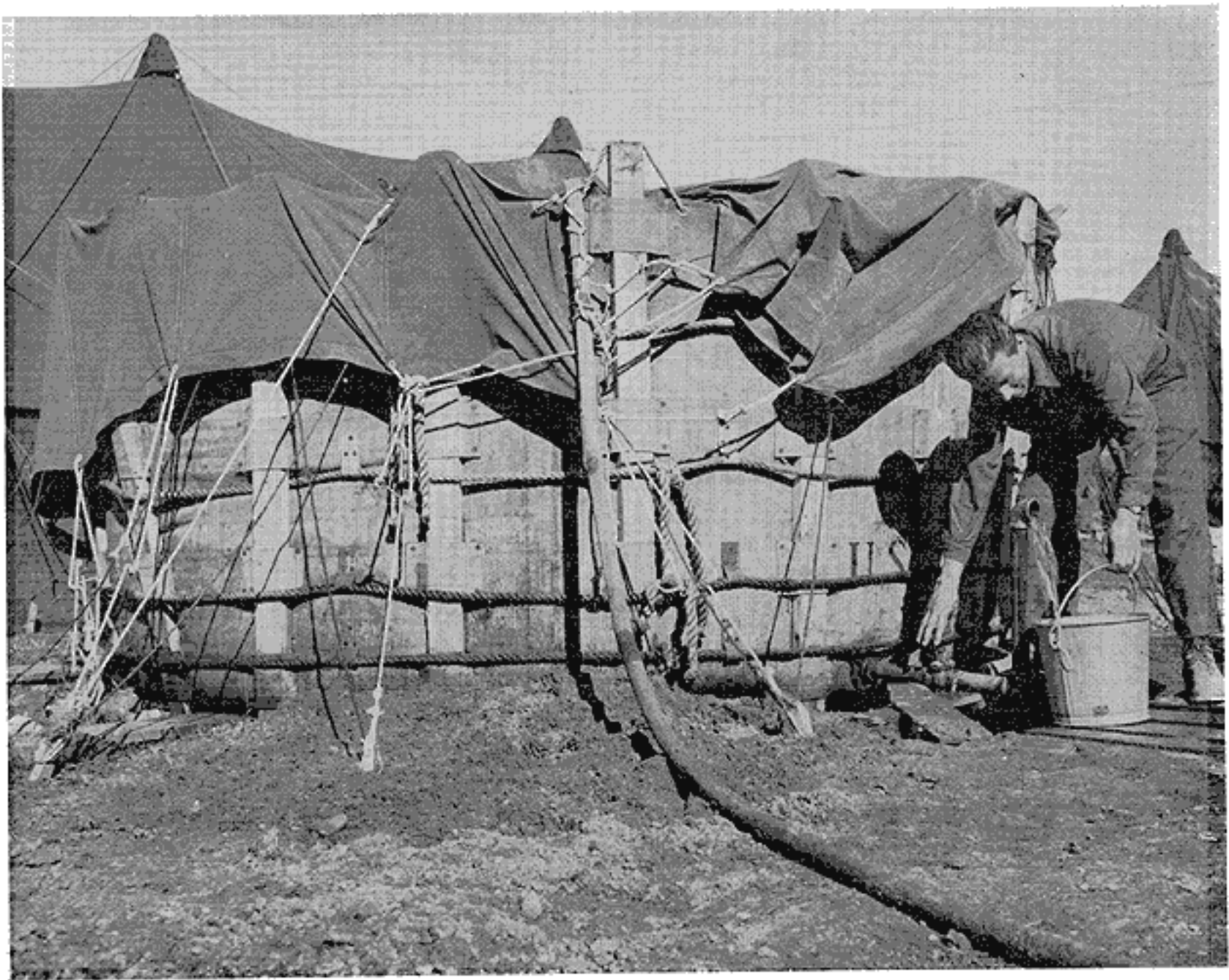
An Army—and particularly an army hospital—requires great quantities of water and often it is obtained with considerable difficulty. The water goes into this 38th tank through the pipeline over the top and comes out the pipe at the bottom.
